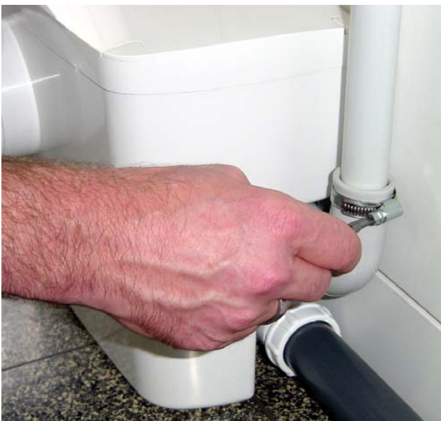
(Pic.4) To connect the pressure hose, please fasten the 1" (DN25) pipe at the outlet bow, which is on the right at the tank of the Saniflux, with a clip. Install the pressure hose upwards (best way: first vertically, than horizontally) in a loop above the sewer level. This will avoid that waste water will flow back into the tank in case excess water (e.g. heavy rain) is in the sewer. Install the pressure pipe directly to the next soil stack. Please check again all connections and make sure that they are sealed. Now connect the unit with the power cable to the main supply and the unit is ready for operation.
