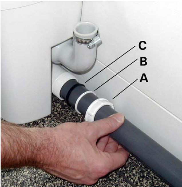
(Pic.3) Put the nut (pos. A), the white plastic ring (pos. B) and the sealing ring (pos. C) onto the DN 40 discharge pipe as shown above and put the pipe into the inlet of the tank. Connect the discharge pipe by tightening the nut to the inlet device. The black sealing ring must be between the nut and the inlet device. Please do the same in case you want to install any additional sanitary units.
