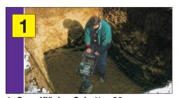
1. Grundfläche: Schotter 30 cm, Sauberkeitsschicht (5 cm Split). Excavate hole and prepare base with compacted gravel.
